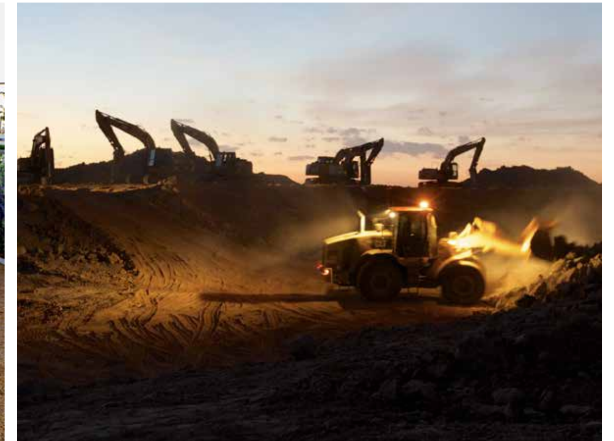
Earthworks & Mass Excavation
